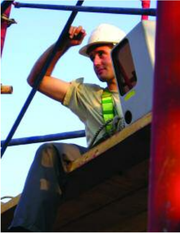
Fig 34 Laser scanning from scaffolding (courtesy of Duncan Lees, Plowman Craven Associates).
