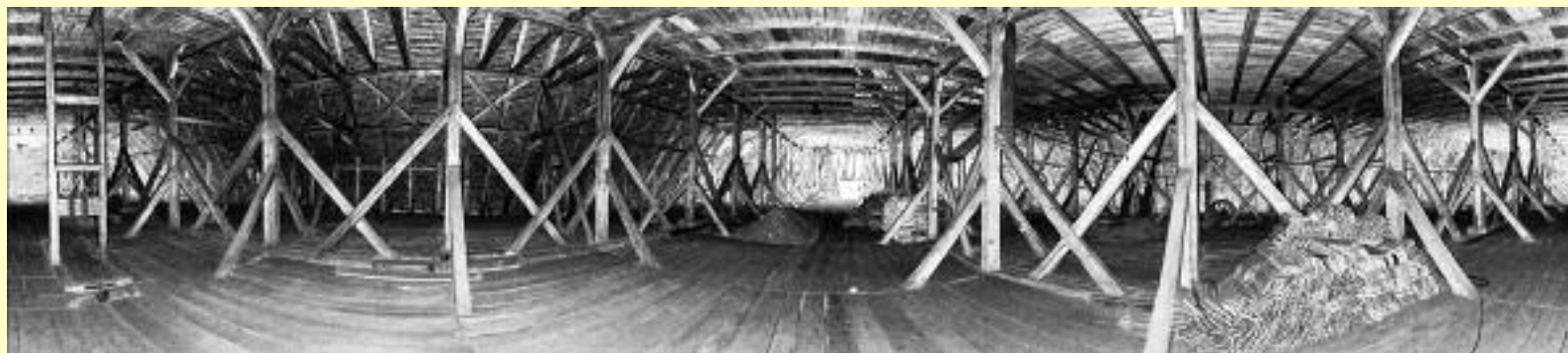
360° x 80° intensity image within the roof truss.
