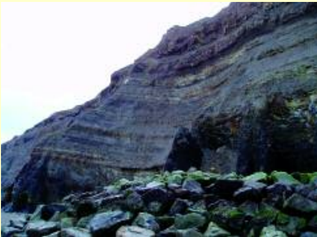
The site is under threat from coastal recession.
